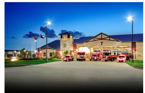
Baytown Fire Station 7
