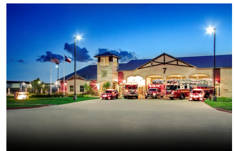
Baytown Fire Station 7
